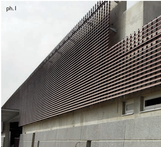
Station épuration - Lattes (34)
